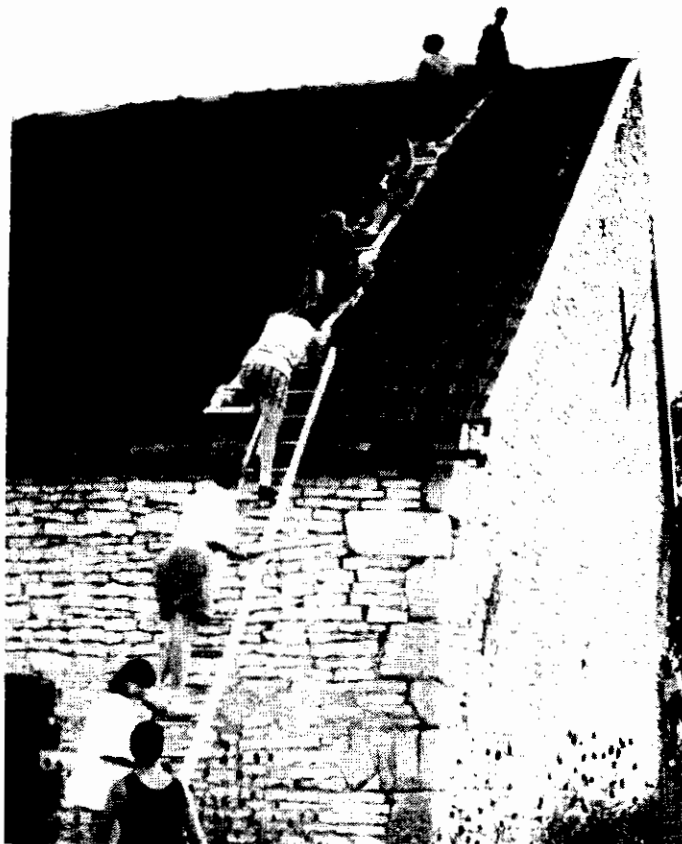
Roofing at Terra Photo by Catherine
