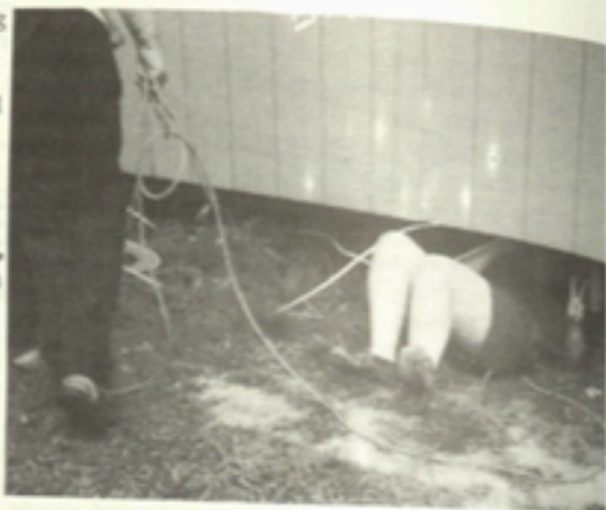
Wiring New Hope Cabin at SUBAMUH. 1997.
