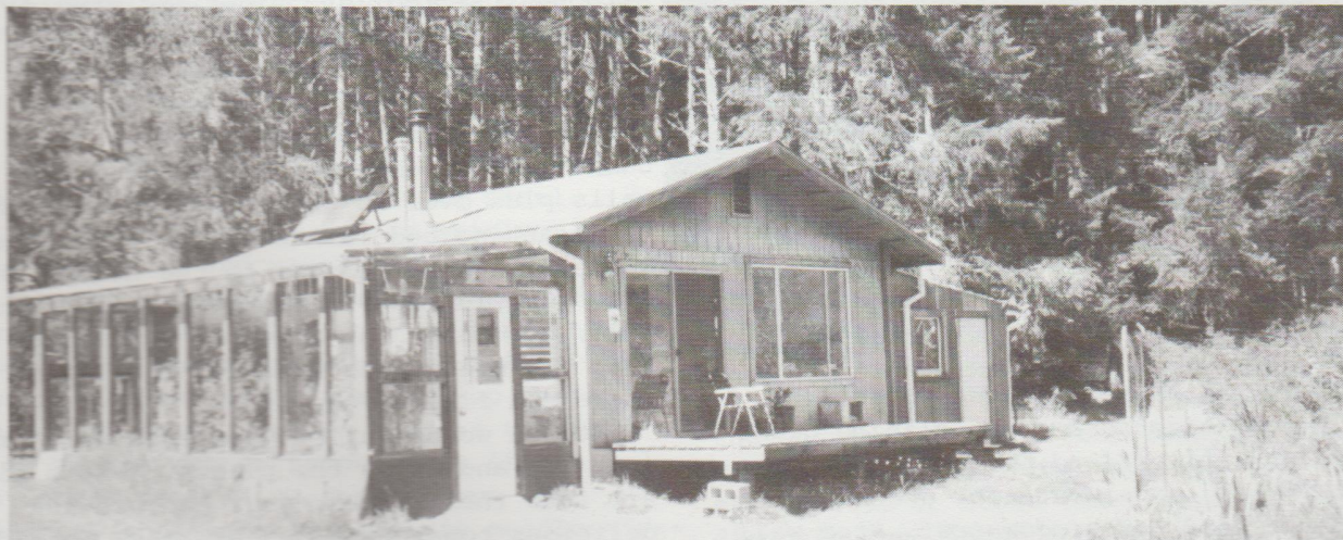
Southeast corner, showing greenhouse, deck and solar water heater on the roof. Spring 1997
