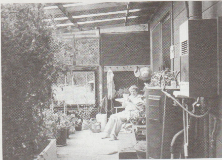
West half of greenhouse interior with terratile floor, tomato vine in planting bed, solar hot water storage tank and back up instantaneous water heater. Spring 97. Photo by Pelican.
